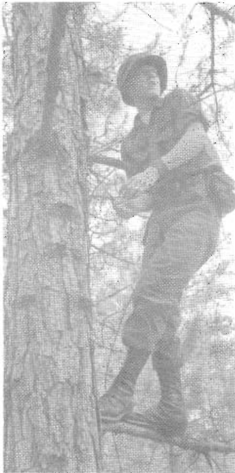
SPEC. 4 RANDY MARSHALL , of Georgetown, a member of Company C, 42nd Aviation Battalion, works in the trees to string communication lines as his unit sets up field operations.
