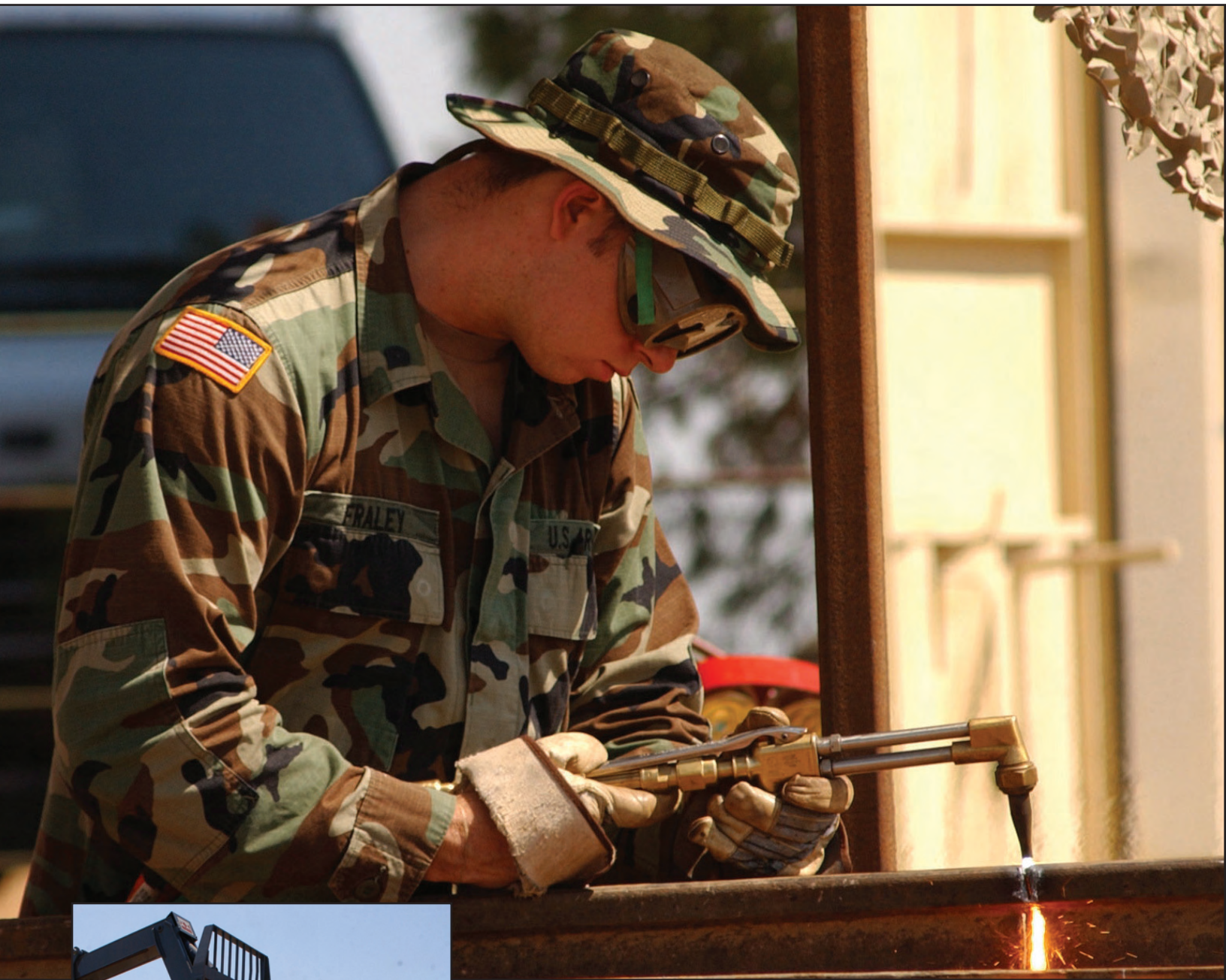
Spec. Tony Fraley, Bravo Company 206th Engineers cuts a steel beam that will be welded into a temporary vehicle barrier in Sasabee Ariz. along the Mexican border.
