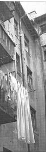
and laundry n, despite the struction.
