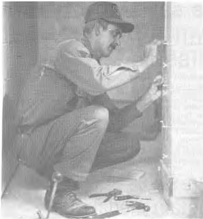
SSgt Robert Richardson installs ceramic tile.
