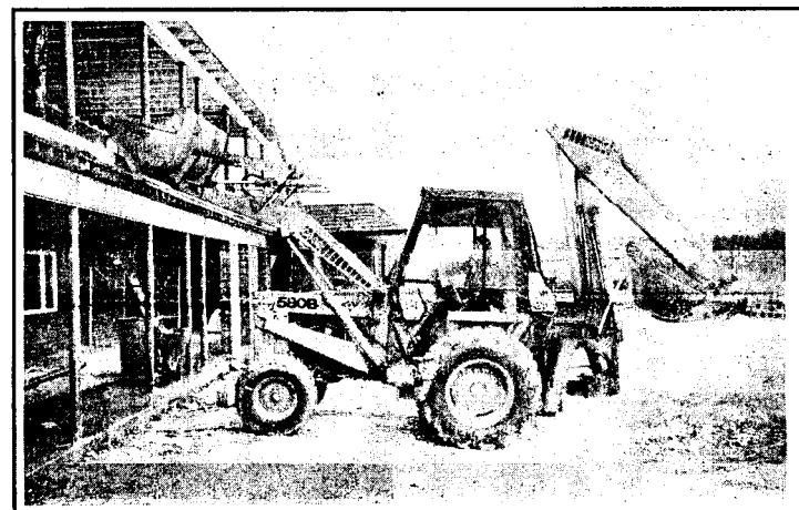
The front bucket of Spec. Charles H. Hannah's backhoe is used to catch waste from the remodeling work on the second floor of the Annex.
