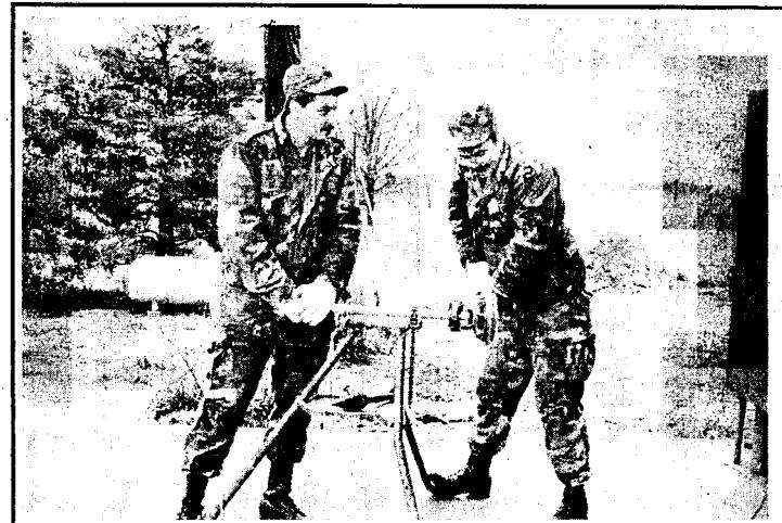
Spec. John E. Stone (right) and SGT Thomas R. McGraw of Headquarters Co., 201st EN BN, thread a conduit for wiring to be used in the Annex.
