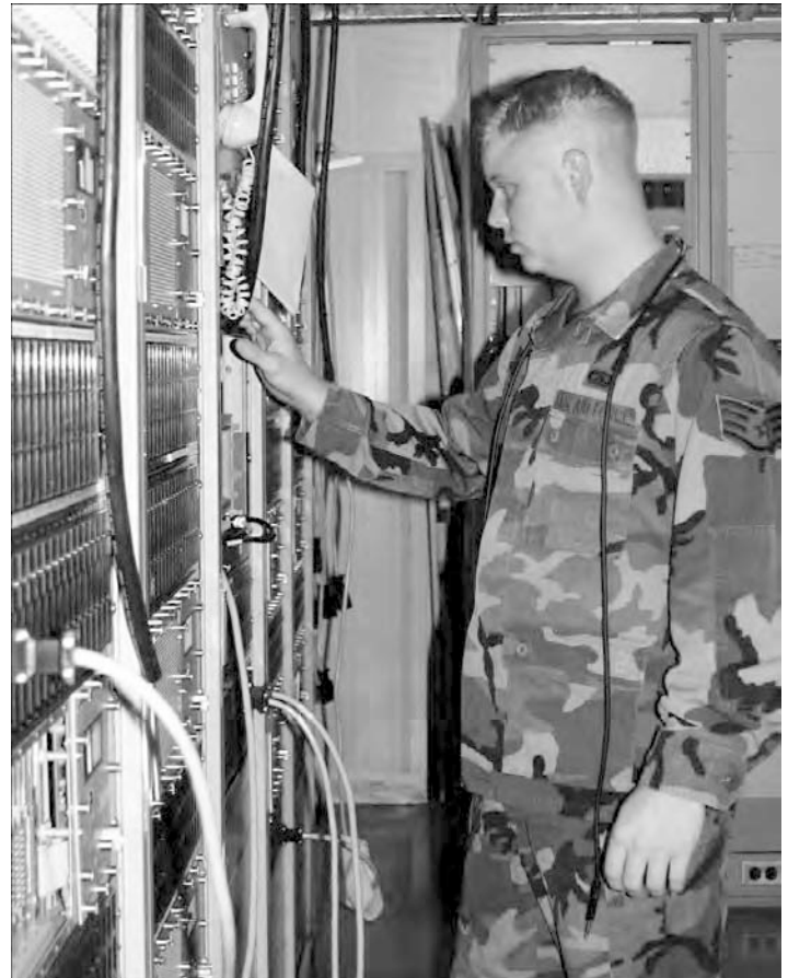
Staff Sgt. Troy Gritton works on a telephone switching panel during a deployment.
