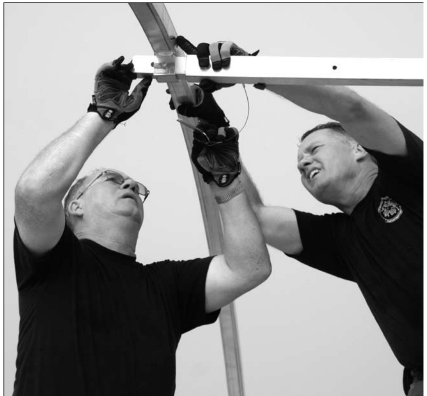
Below: Tech. Sgt. Gary Risen and Lt. Col. Bill Adkisson of the 123rd Medical Group connect beams used in the support structure of EMEDS facilities.
