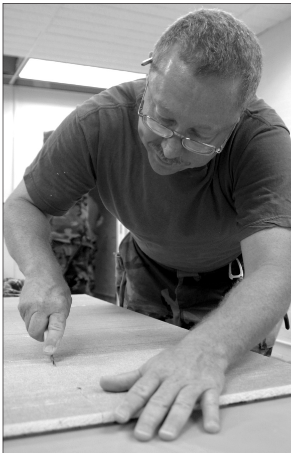
Above: Master Sgt. Larry Broyles trims ceiling tile during a facilities upgrade at the Mintos Armory.
