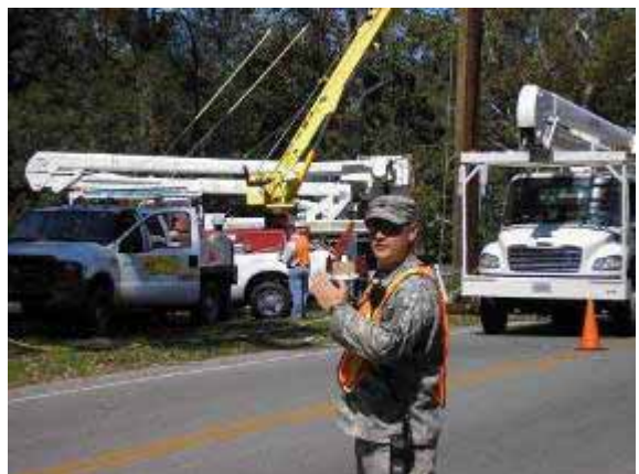
SGT Desha of Co B, 351 st ASB directs traffic around power lines destroyed by Hurricane Ike after it skirted Louisville, KY.
