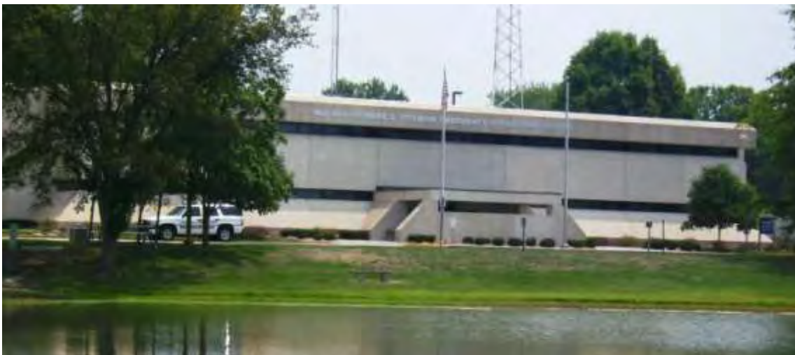
Maj. General Richard L. Frymire Emergency Operation Center, Frankfort, KY
