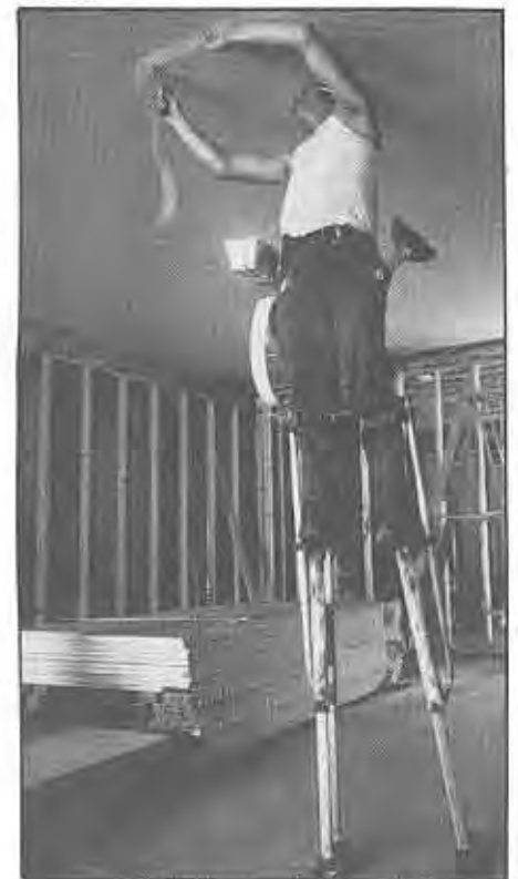
KyANG Photo by A1C Dennis Robinson Sgt. Michael Mudd, 123d CES Taping drywall using stilts
