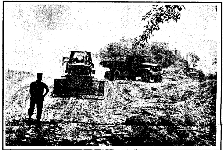
SGT Tim Tucker dozes dirt into place over a culvert installed by the engineer company.
