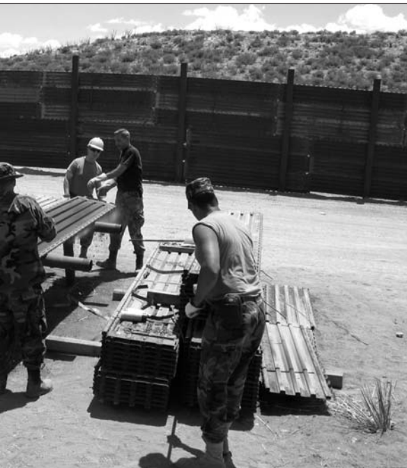
Workers weld pieces of steel matting together near
