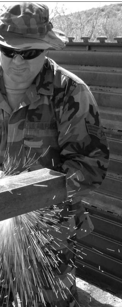
Left: Senior Airman Mike Ferris of the 123rd Civil Engineering Squadron cuts steel beams used in the construction of fencing along the U.S.-Mexican border.
