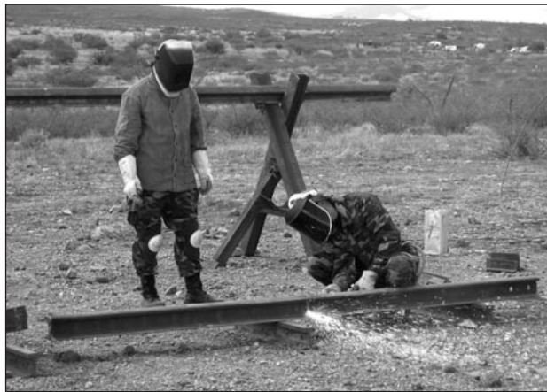
Left: Senior Airman Mike Ferris of the 123rd Civil Engineering Squadron cuts steel beams used in the construction of fencing along the U.S.-Mexican border.
