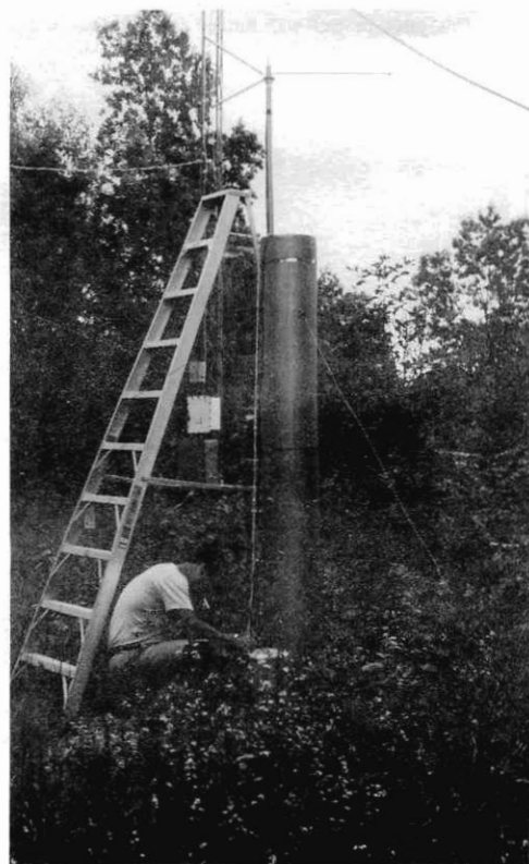
DES TECHNICIAN JOHN SEMONES installs monitoring equipment associated with the Radio Reporting Rain Gauge Program in Eastern Kentucky.
