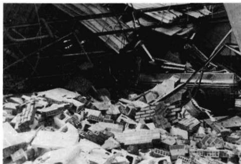
A TORNADO hit Winchester June 16, 1982, demolishing a tire store while it cut a two-mile swath along U.S. 60.
