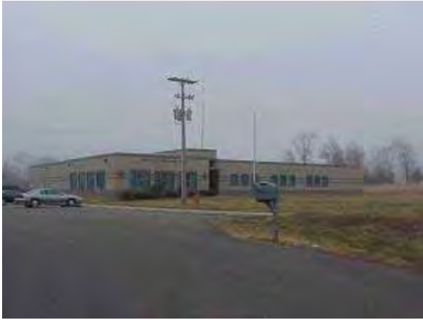
Leitchfield Readiness Center
