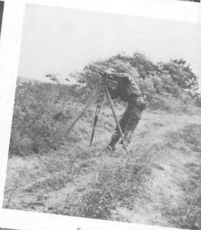
Surveying for a bridge.
