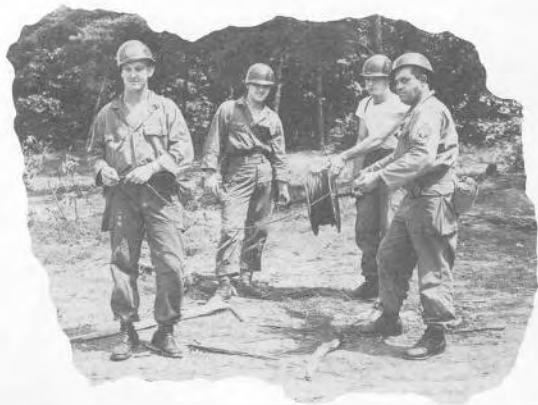
Stringing communication lines.
