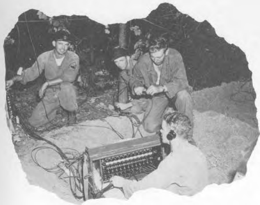
Setting up the switch board center.
