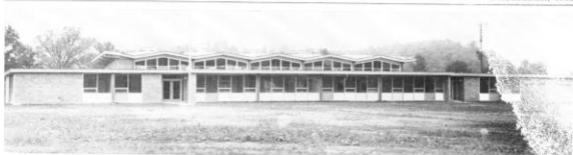
New Barbourville National Guard Armory
