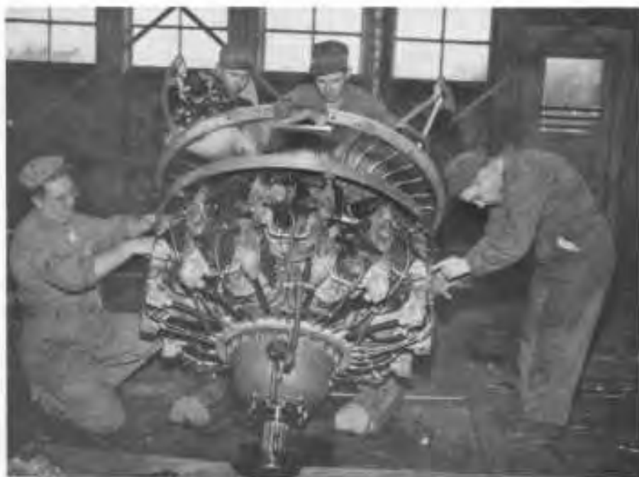
ENGINE REPAIR: Even a C-47 engine has to be pulled sometime. Working on this Pratt & Whitney radial were (from left) Ralph Bronget, George Heim, Willie Goatley, and Herbert Settle. Note those grease-monkey coveralls.
